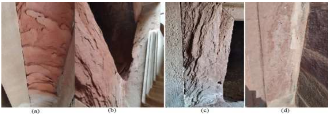
Fig. 2 (a), (b), (c), and (d) Deterioration of sandstone in Khusro tombs structure
